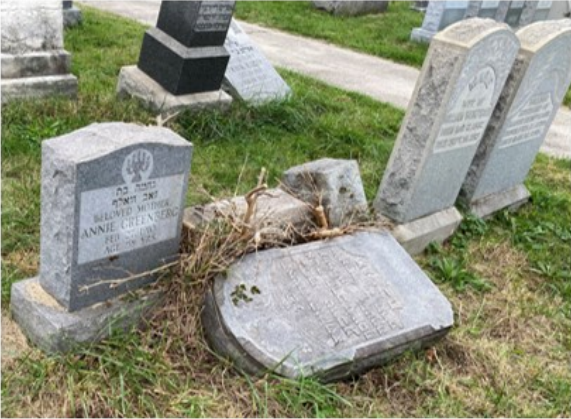
From fallen, leaning, and at risk.
